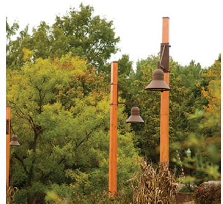
Light source shielded to avoid glare
